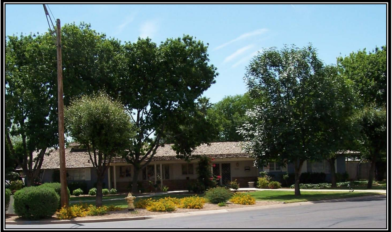
5737 West Royal Palm Road Photo: Glendale Planning Department
