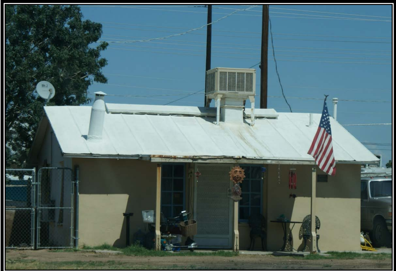
Typical Adobe House
