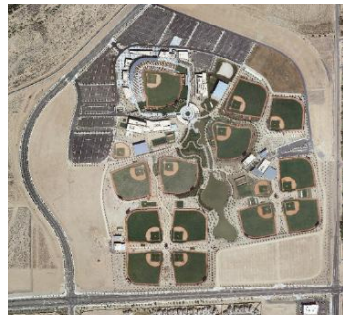
From farm fields to ball fields in just over 15 months of construction time.
